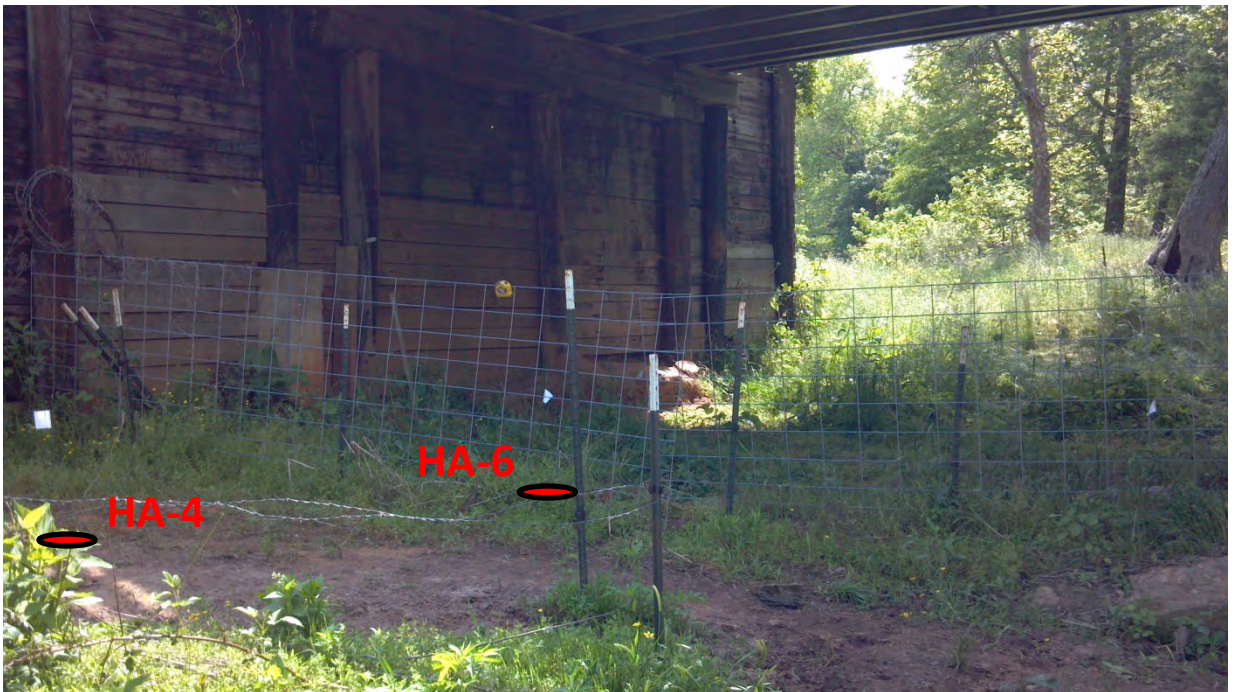
Photo #6: Locations of HA-4 and HA-6 advanced on the eastern side of the northern bent. The photo was taken from the south looking north.
