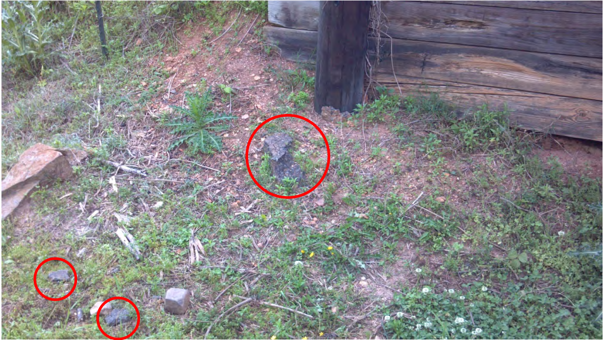
Photo #8: Asphalt pieces observed on the ground surface adjacent to the northern wing wall.
