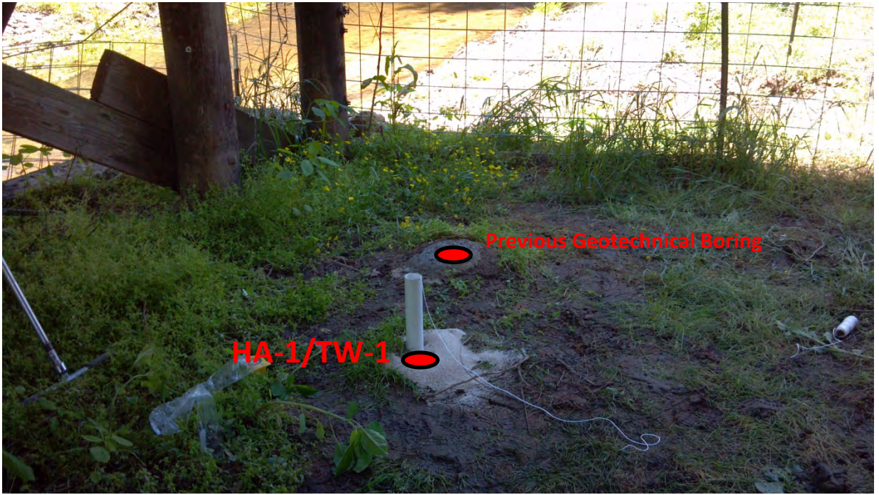
Photo #2: Location of HA-1 which was converted to TW-1. The previously advanced geotechnical boring can also be seen. Photo was taken from the northwest looking southeast.
