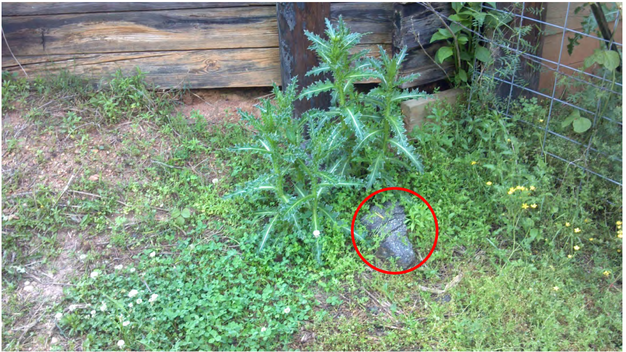
Photo #7: Asphalt pieces observed on the ground surface adjacent to the northern wing wall.
